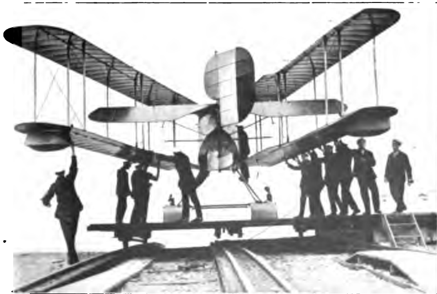
A British Seaplane with Folding Wings
